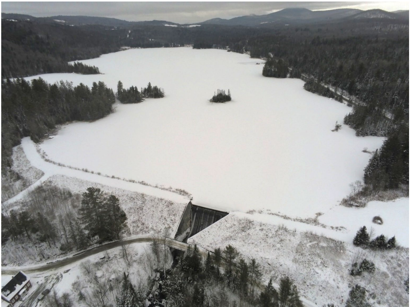
Figure 16: Thurman W. Dix Reservoir Dam in Orange
