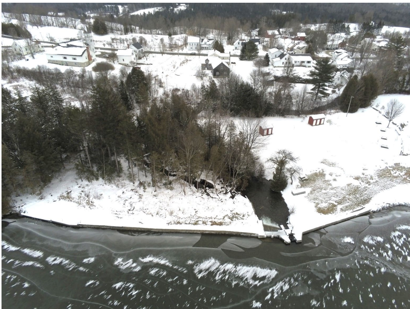
Figure 17: Caspian Lake Dam in Greensboro
