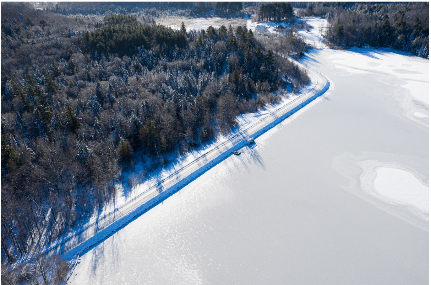
Figure 18: Kent Pond Dam in Killington
