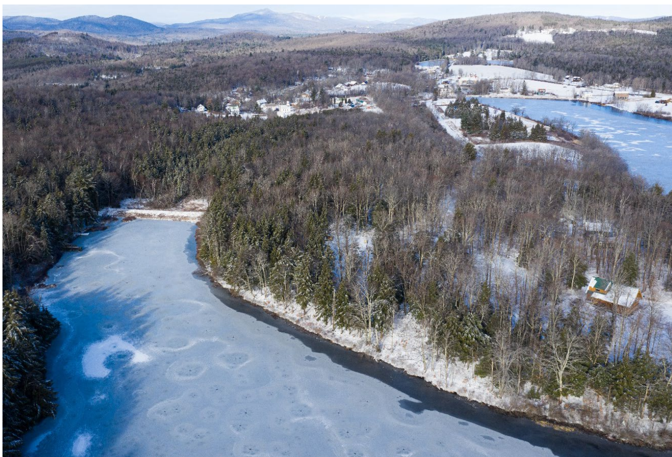
Figure 15: Lake Sadawga West Dike in Whitingham
