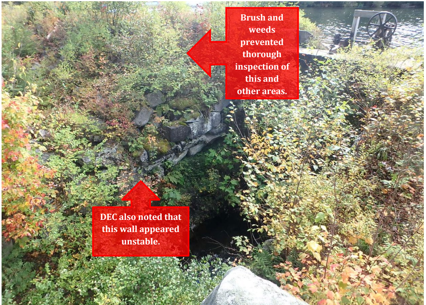
Figure 7: Brush and Weeds Around a Portion of East Long Pond Dam in Woodbury, Vermont a
