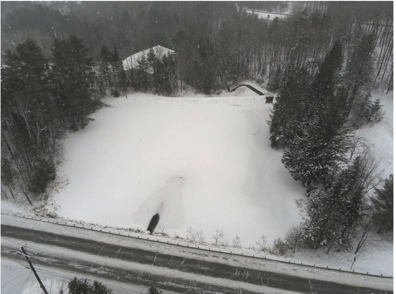
Figure 11: Institute Pond Dam in Lyndon
